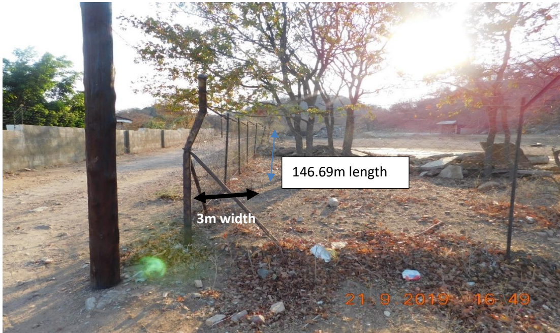
Western edge of commercial plot of PAP 1, which abuts an existing access road showing existing fence to be moved. 220.042m 2 (3m width x ~146.69m length) 3 of land is to be acquired and two trees to be cut. The area to be acquired will not impact economic activity resulting in disruption of livelihoods. However, this was subsequently changed in February 2020 to 1.5m following construction by the PAP who left a 2.2m distance. See Plate 1b.
